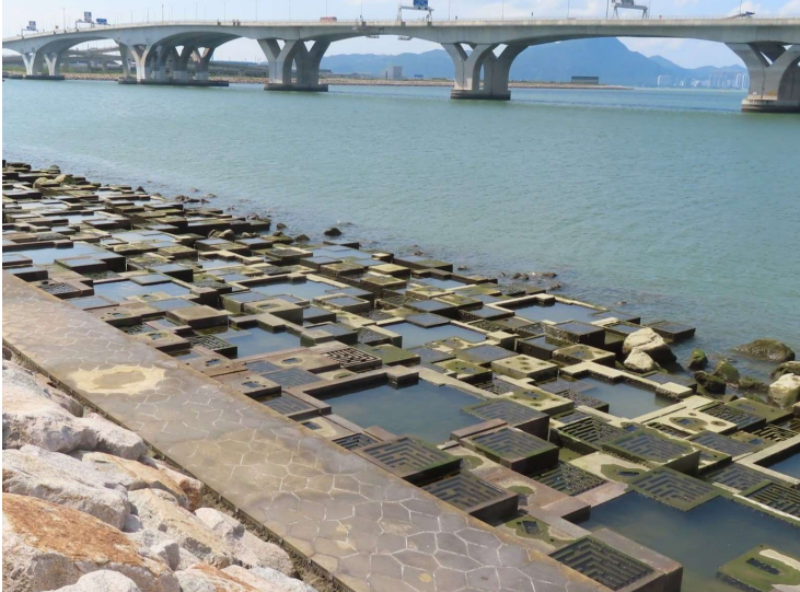
General View of Rocky Eco-shoreline
